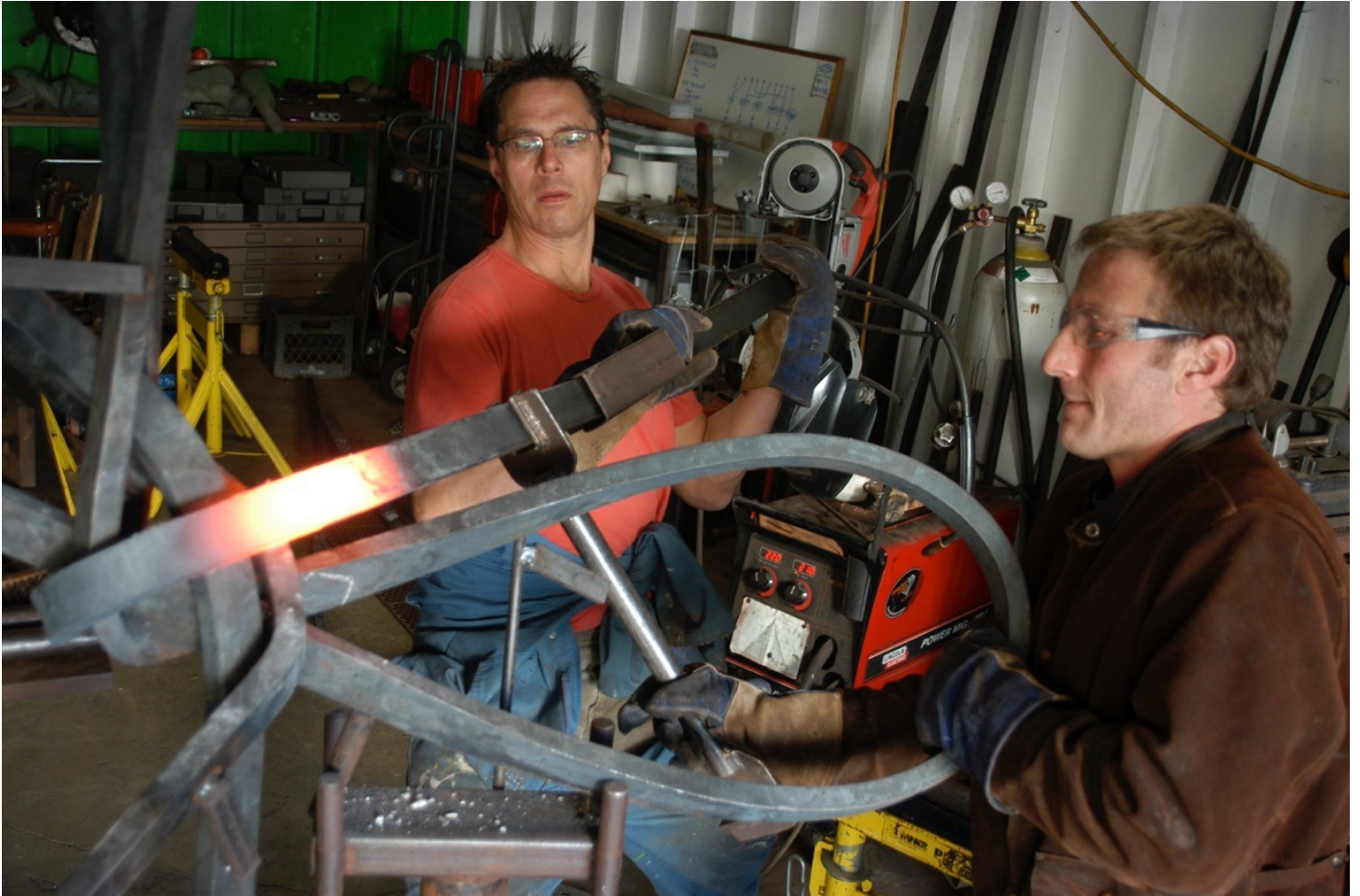
Schifrin and Duskin work together while forging hot steel for the project. Photo courtesy of Peter Schifrin.
